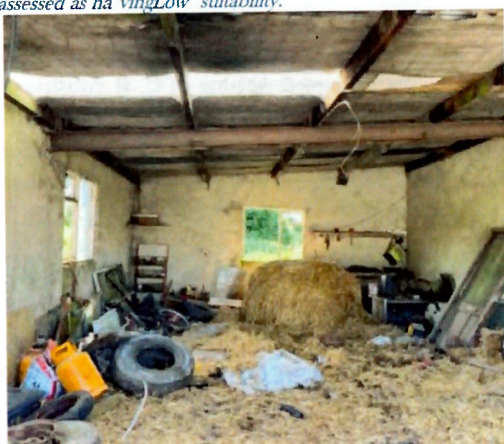
Plate 4-17 Felt underlining in open-fronted shed.
