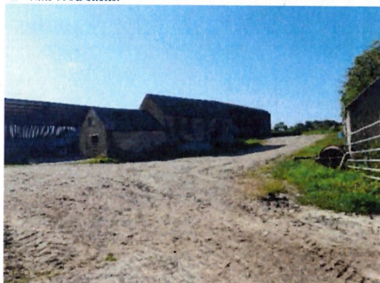
Plate 4-7 East aspect of western shed.
