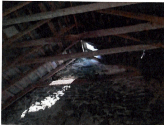
Plate 4-24 Felt underlining and damaged roof offering access and roosting potential for bats.
