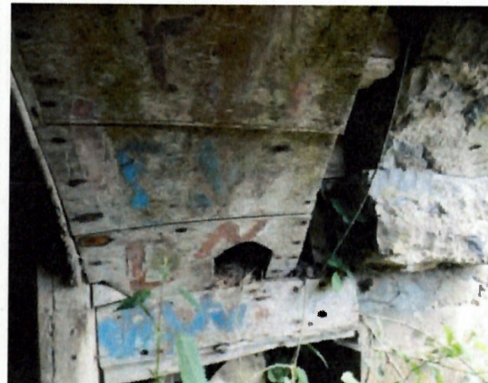
Plate 4-14 Internal stonework of western shed.
