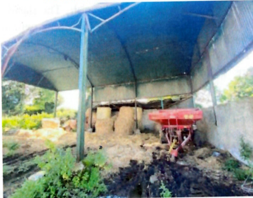
Plate 4-27 Another galvanised metal shed.
