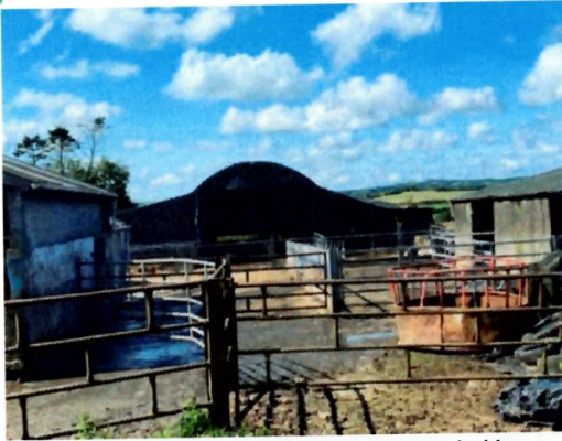
Plate 4-25 Galvanised metal sheds assessed as Negligible.
